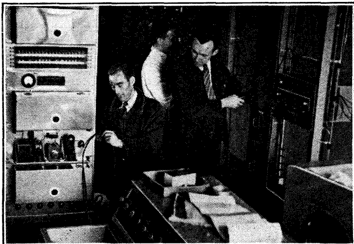
NEW CENTRAL CONTROL ROOM, which is nearing completion at Alexandra Palace, will be the nerve-centre of television broadcasts. It will handle the outputs from the two studios as well as those coming from the O.B. units.
